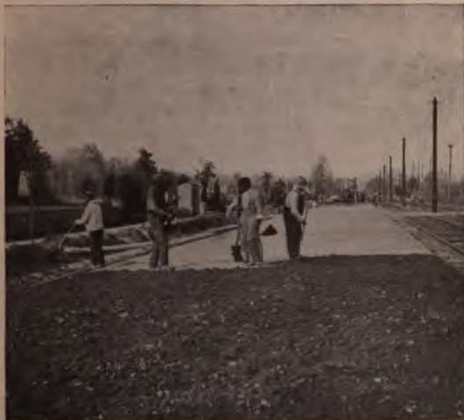
Covering With Earth.
